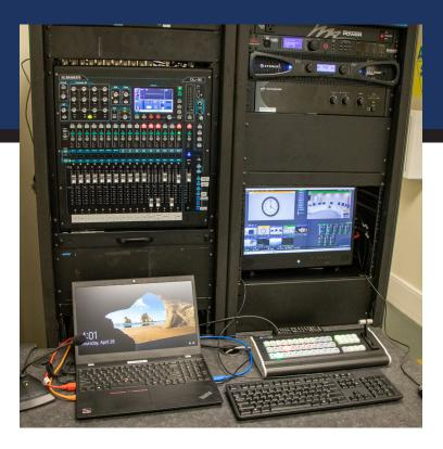
Currently, they're taking the traditional route to control cameras through vMix in pop-up windows to control their presets. They are still waiting on two vMix machines to be delivered (integration from a company called Acme Video Solutions), essentially all-in-one machines that run vMix as the digital switching software and has AJA, SDI input cards, board panel controller, two lines program preview, and a T bar to transition between. This eliminates the need for a dedicated streaming PC.
